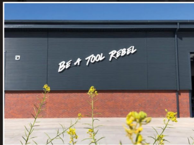
Wera distribution centre Large commercial unit
